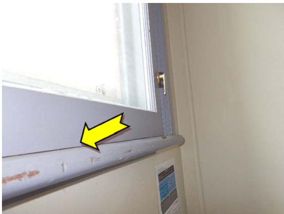
Photo 17. Interior, staircase, skirting and window frames – suspected lead-containing light purple upper paint systems.
