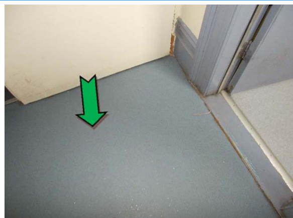
Photo 6. Interior, ground level, east elevation, adjacent small preschool room, blue floor coverings – non asbestos-containing sheet vinyl.
