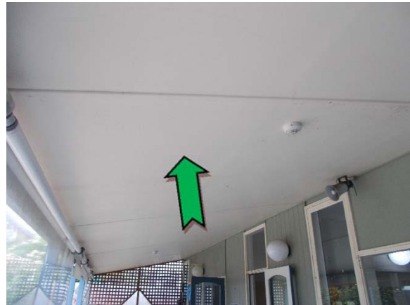
Photo 4. Exterior, ground level, south elevation, awning – non asbestos-containing fibre cement sheeting.
