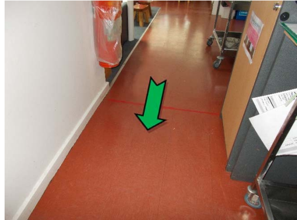
Photo 8. Interior, ground level, large preschool room, red floor coverings – non asbestos-containing vinyl floor tiles.
