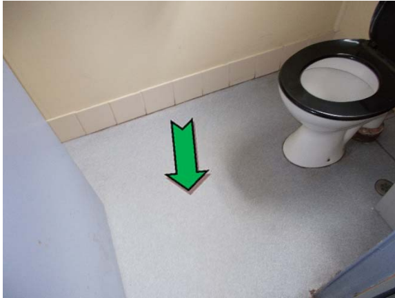
Photo 7. Interior, ground level, east elevation, toilet, light blue floor coverings – non asbestos-containing sheet vinyl.
