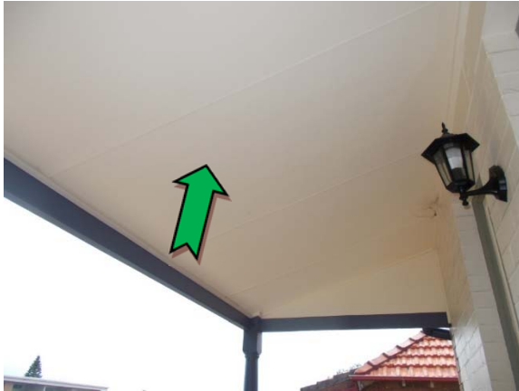
Photo 1. Exterior, level one, north elevation, awning – non asbestos-containing fibre cement sheeting.
