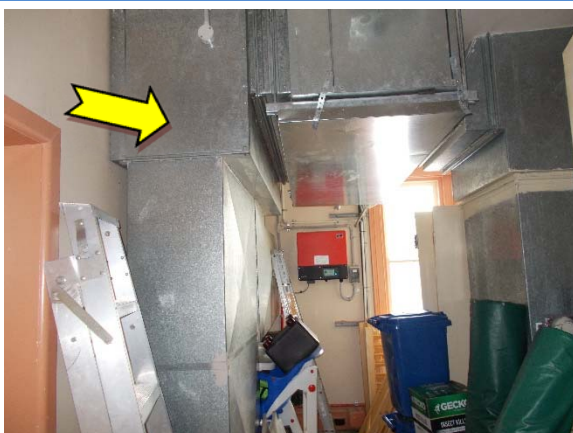
Photo 11. Interior, level one, throughout, ductwork – suspected SMF internal insulation material.
