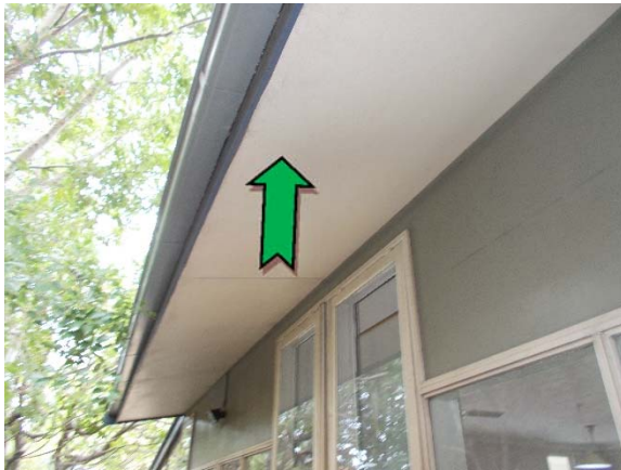
Photo 3. Exterior, ground level, south-east elevation, eaves – non asbestos-containing fibre cement sheeting.
